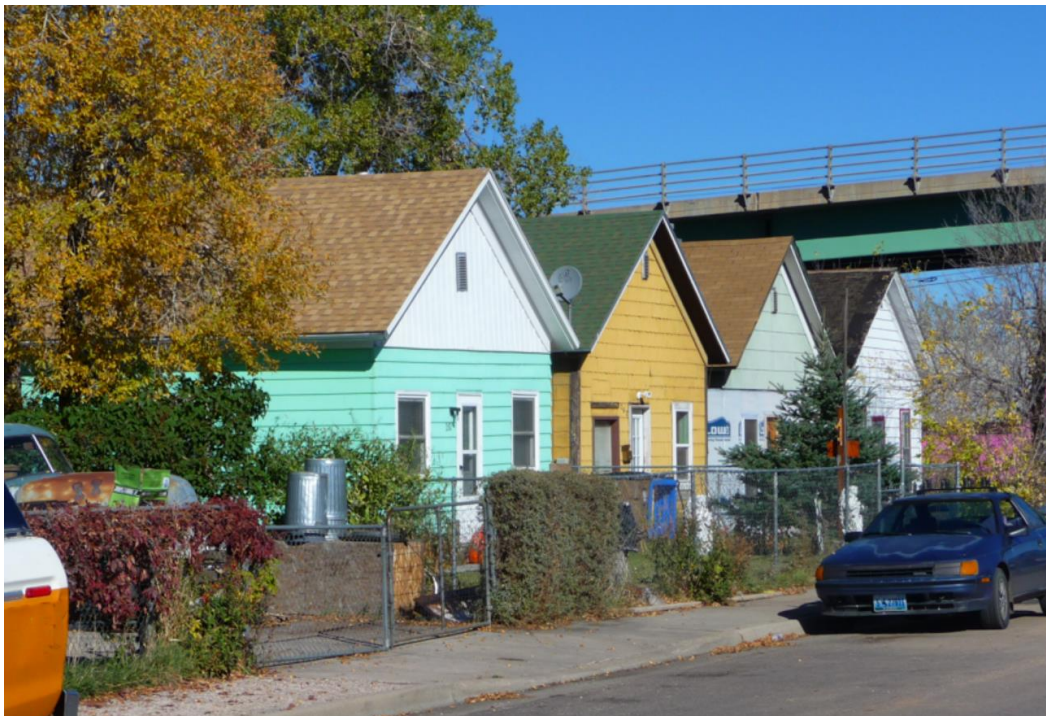
Figure 2 - Row of houses built by the Union Pacific, Photograph by Mary M. Humstone, SAH Archipedia
