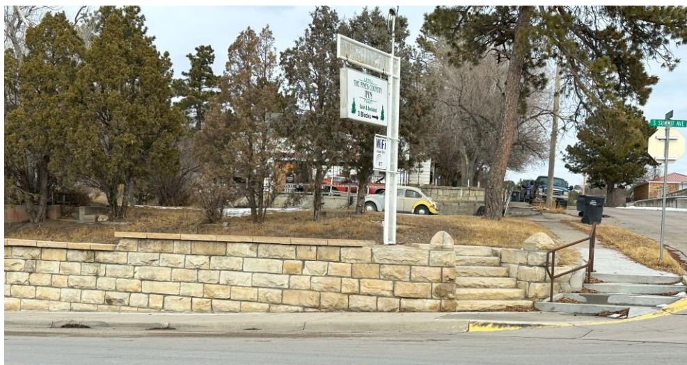
Figure 27 - Example of Repaired Retaining Walls in Newcastle, Photo by Author
